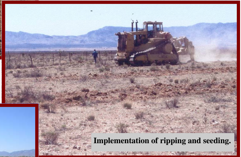
Ripping and seeding area after treatment.
